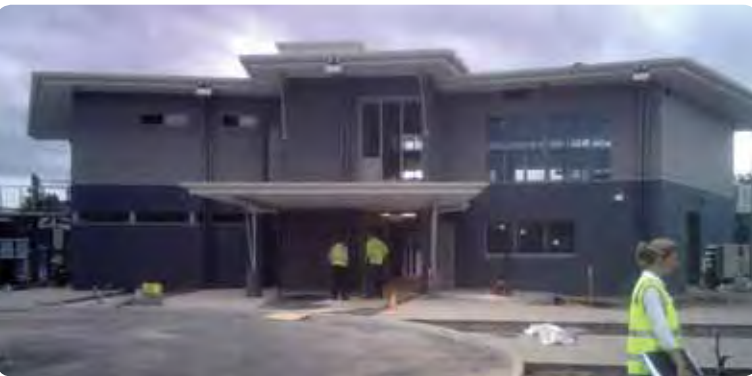
A site inspection was conducted in 2010.
